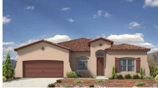
Victoria Mission Tile Roof
