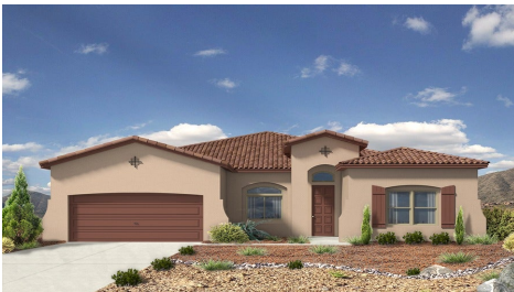
Victoria Mission Tile Roof
