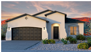
Tabitha II Mission Shingle Roof
